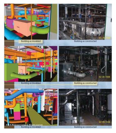
Figure 42: A coordinated composite 3D model of the various MEP systems resulted in high degree of fabrication accuracy and simplified error free installation (Mortenson, 2009).
