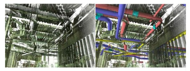
Figure 25: Left: result from laser scanning. Right: Model superimposed on the laser scan to validate as-build accuracy (SMCCV website, accessed on Oct. 2011)
