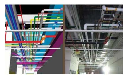
Figure 46: MEP Coordination and field verification by Mortenson resulted in an as-built facility that is very close to as-planned. (Mortenson 2009)
