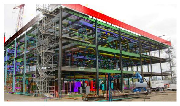
Figure 37: Photo-match of 3D Model to Construction Progress - Feb. 2010 (Ghafari Associates, accessed on Oct. 2011)
